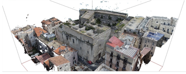
(a) Aerial view.
